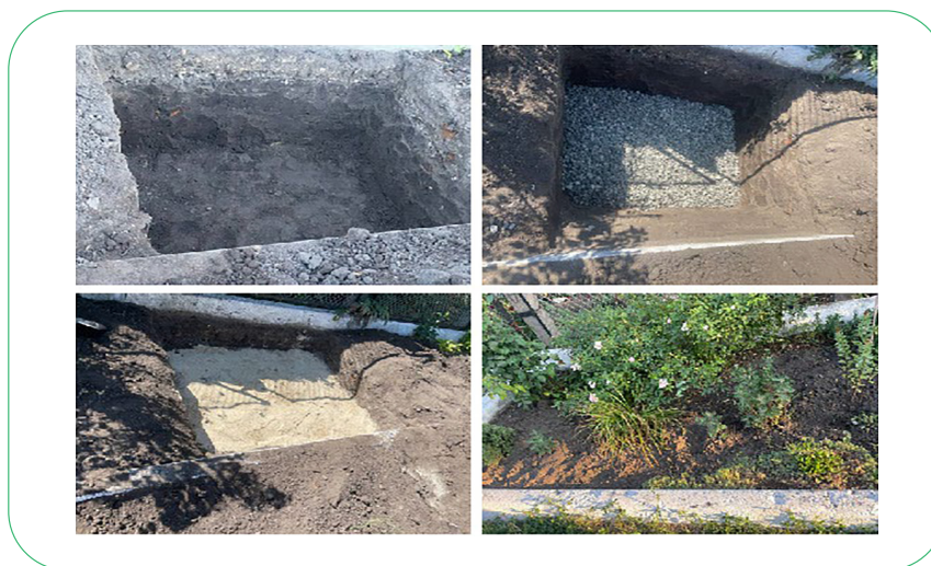
Figure 1. Construction stages of the RG (Kyiv region)
